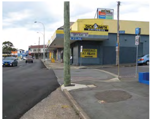
At Tighes Hill commercial centre on Maitland Road street tree planting is constrained by overhead services and awnings.
