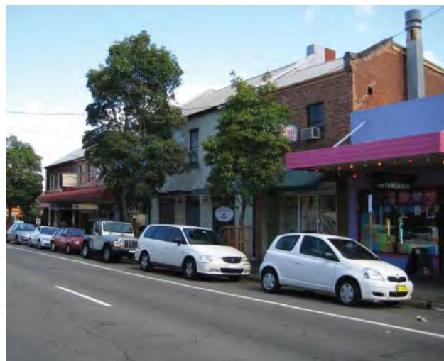
Darby Street is a busy commercial centre planted with Brush Box street trees. Power lines have been bundled.
